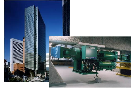
Seismic Isolated Building (Japan)
