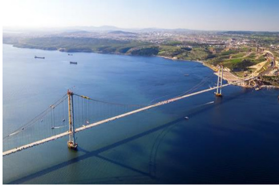
Osman Gazi Bridge (Turkey)
